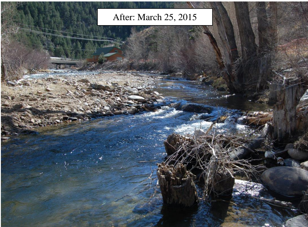
Figure 1.6. Post-construction photo of the downstream “low-intensity” stream site (side-channel treatment) as part of the Twin Tunnels project on Clear Creek.
