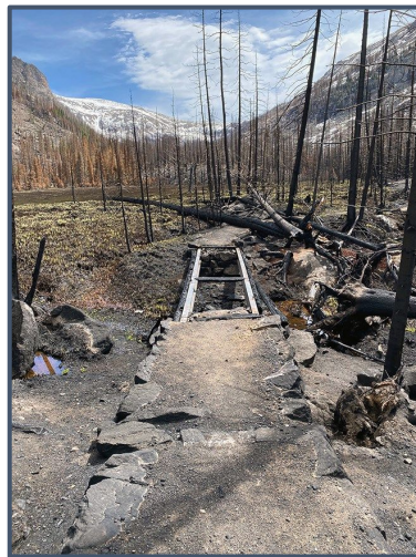
Photo: NPS Footbridge along the Tonohutu Trail after the East Troublesome Fire
