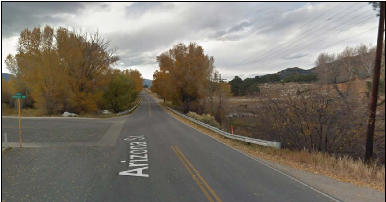
Photo 1 - Northern Terminus of County Road 313 Trail looking north at intersection of Arizona Street and Marquette Ave shows existing Cottonwood Creek vehicle bridge
