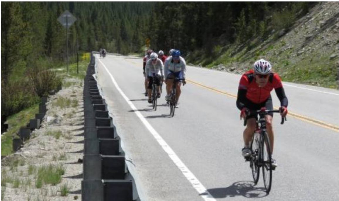
Cyclists and heavy vehicular traffic must share eleven foot wide traffic lane, steep grades, and limited shoulder width through “the narrows” on State Highway 91.
