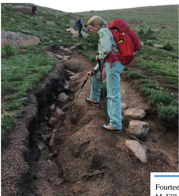
Fourteener Program Manager Loretta McEllhiney points out sections of trail suffering from erosion, resulting in deep gullies that increase destructive water flow. The gullies also cause hikers to step off the trail, further exacerbating the problem. *Photos by Emily Olsen, NFF*
