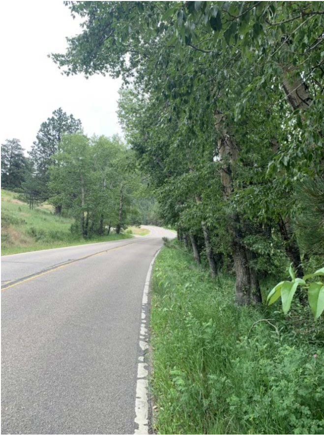
Figure 4: there is no shoulder along Fish Hatchery Road on either side as the road approaches US34
