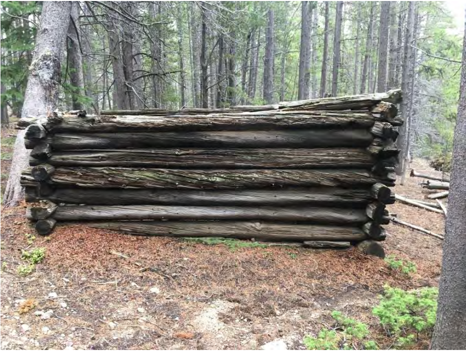
Log Cabin Site
