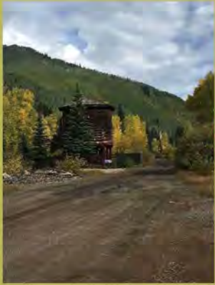
R.G.S. WATER TANK
