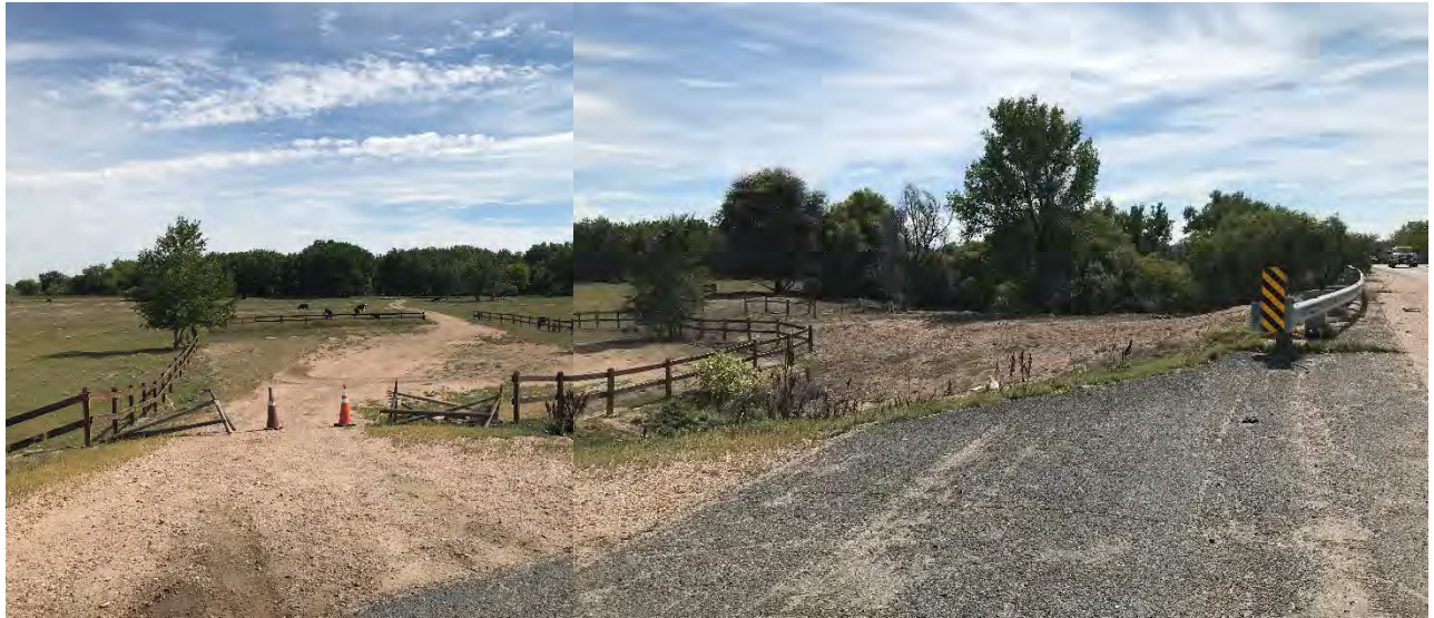
Looking southeast. Fenced area is former oil/gas tank battery site removed in 2018. Trees on right are along the river. If selected, a bridge crossing would need to be installed about 600 feet downstream of the road bridge.
