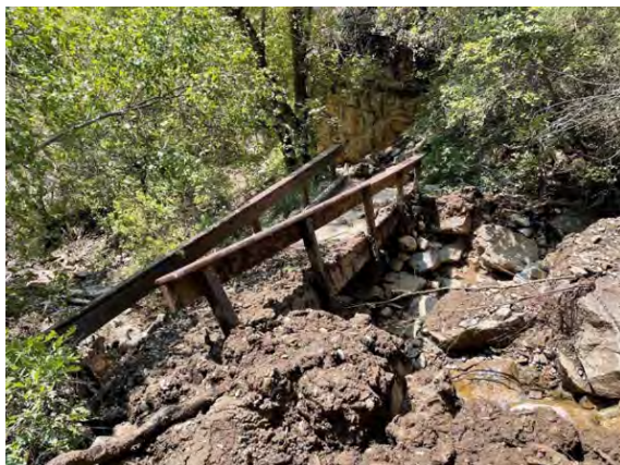
Remnants of Bridge #1
