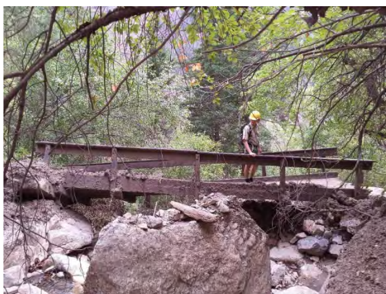
Looking downstream at Bridge #1
