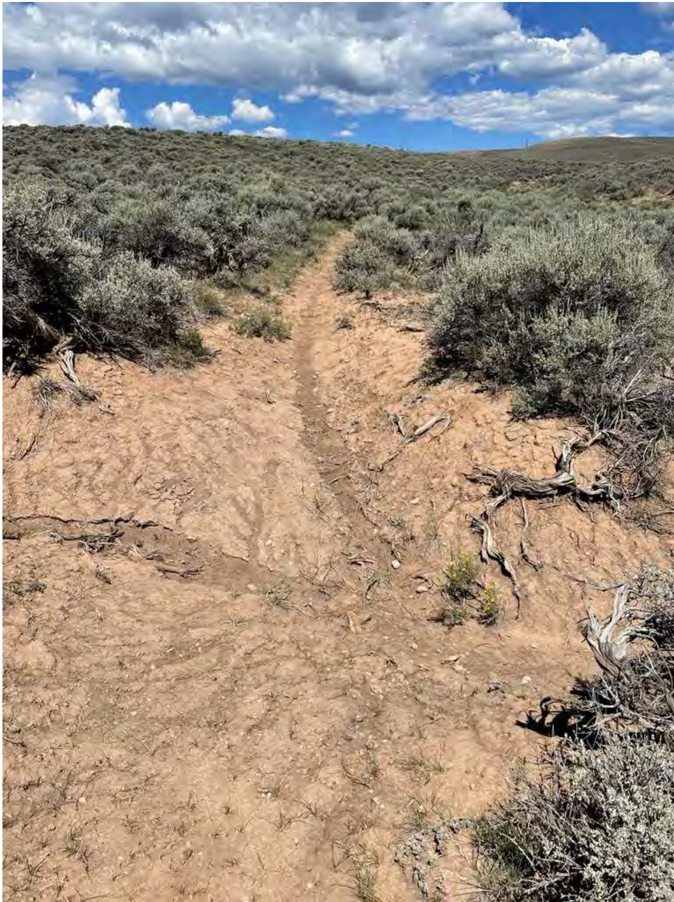
Erosion on the Beaver Creek Trail in need of check steps and drains.
