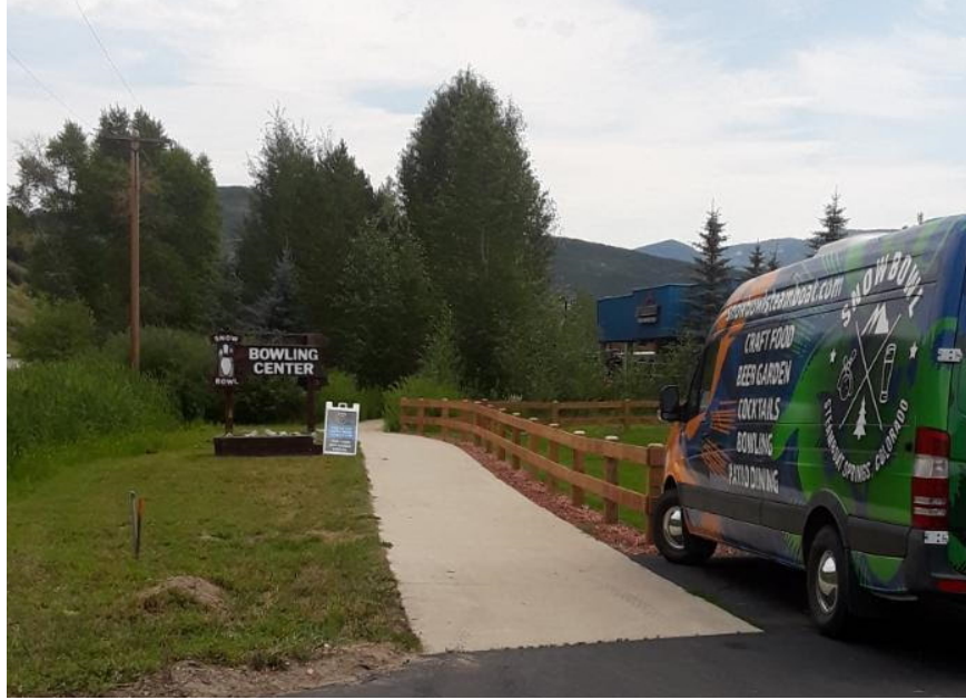
Above Photo shows the current terminus to the Yampa River Core Trail / Sidewalk at the Bowling Alley.
