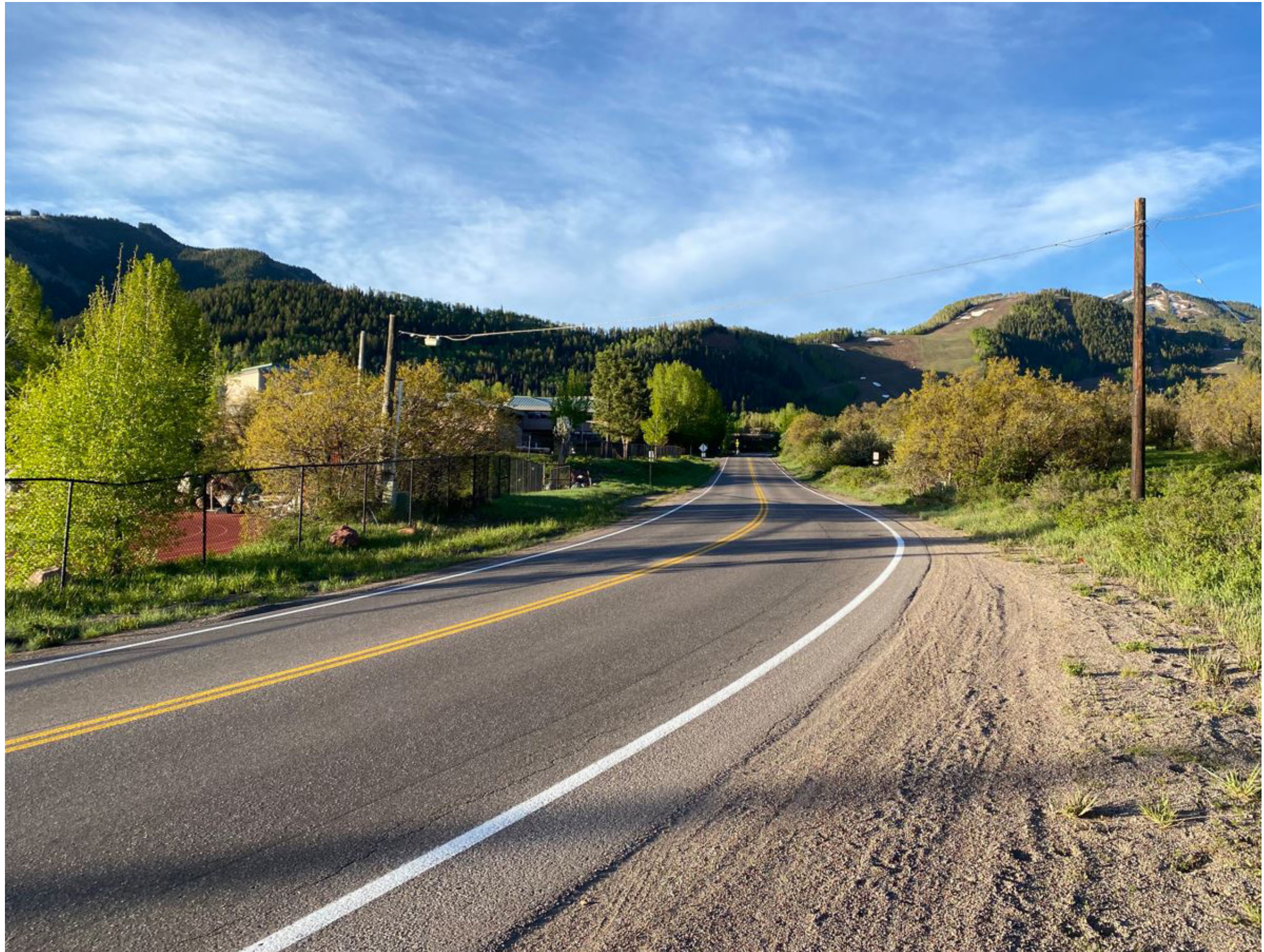
MAROON CREEK MULTI USE TRAIL: SITE PHOTO LOOKING SOUTH MAROON CREEK ROAD
