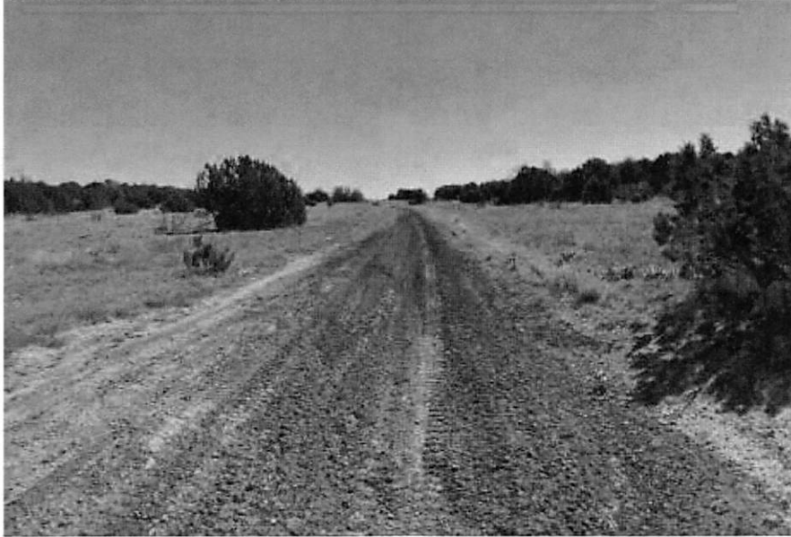
Section of trail at Penrose Commons that had been severely rutted, now rehabilitated with the RRMMC trail dozer.
