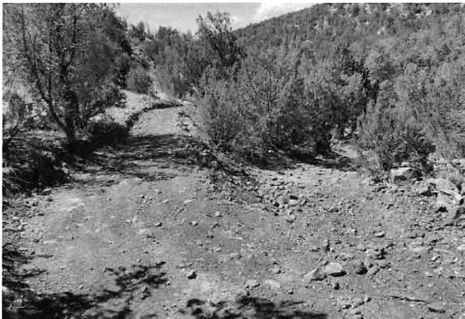
Section of trail at Penrose Commons that had been severely eroded, now rehabilitated with the RRMCM trail dozer and water diversion added to mitigate future damage.
