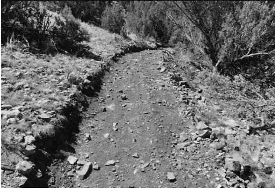
Section of trail at Penrose Commons that had been severely eroded, now rehabilitated with the RRMCM trail dozer.
