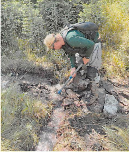
Improving drains and armoring tread
