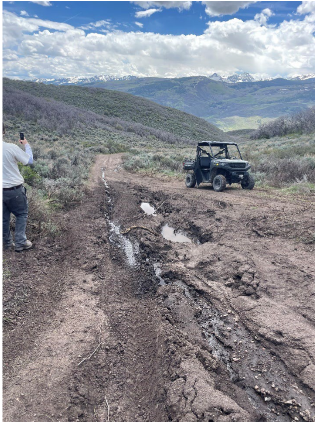
May 2023 - Road damage on the Crown Special Recreation Management Area before OHV Crew maintenance. Damage (photo above) is causing trail braiding by OHV users.
