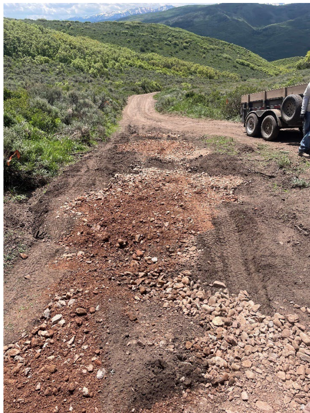
June 2023 - Road damage after OHV crew worked to provide initial maintenance to reduce resource damage. Additional, more involved road maintenance is planned for 2024.
