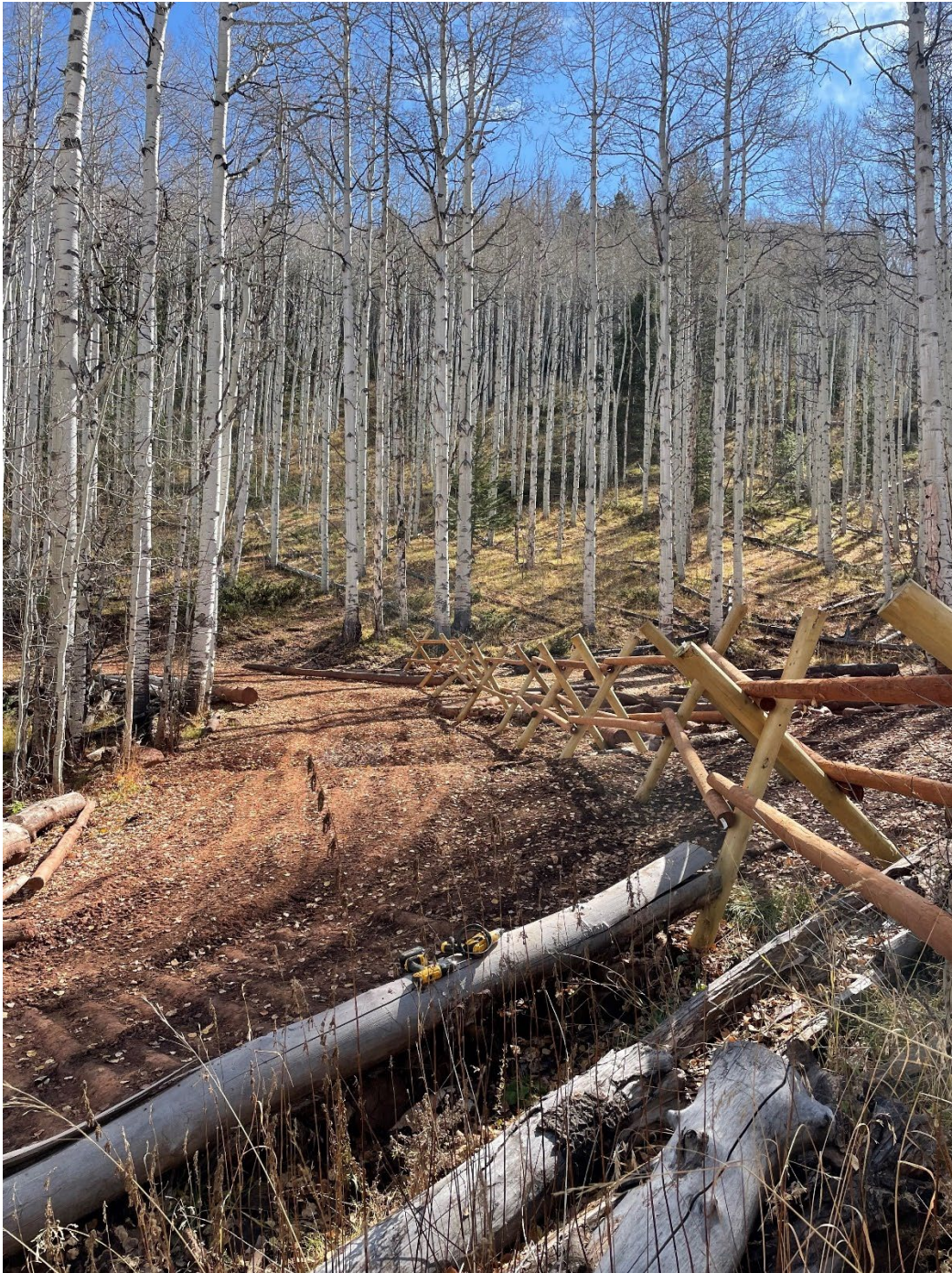
October 2023 - The OHV Crew completed a fence install within the Hardscrabble – East Eagle Special Recreation Management Area (SRMA). The fence will help to encourage OHV users to stay on the designated route and allow for vegetation to reestablish itself in disturbed areas outside of the approved route corridor.
