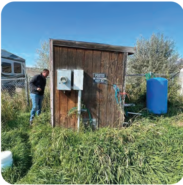
Irrigation Pump House
