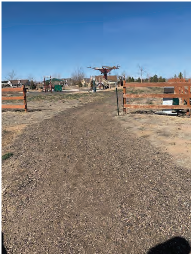
Concrete will change entrance to ADA accessible
