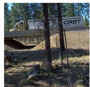
Gilchrist Underpass Wildlife Directional Fencing Project Leader: Oregon Hunters Association Amount: $70,000 Total project cost: $1,000,000 Partners: Oregon Department of Transportation, Rocky Mountain Elk Foundation, Mule Deer Foundation, Oregon Wildlife Foundation, US Forest Service - Deschutes NF, Oregon Watershed Enhancement Board, National Fish and Wildlife Foundation, Oregon Department of Fish and Wildlife, Protect Animal Migration, Oregon Department of Forestry, Coastal Farm and Ranch Location: East Cascades Oregon Hunters Association, the Oregon Department of Transportation (ODOT), and many other partners will install the directional fencing needed to guide animals to the newly constructed Gilchrist Wildlife Underpass along Highway 97. ODOT chose to construct the underpass as an opportunity to replicate the wildlife passage success of the 2012 Lava Butte underpass. ODOT was not able to fund the necessary directional fencing to make the underpass an effective migratory barrier solution. The benefits of barrier-free, animal passage include reducing wildlife loss, economic loss from animal/vehicle collisions and less human injury or death.
