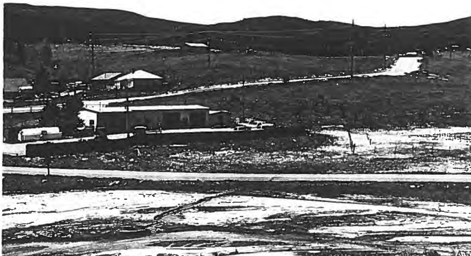
Figure 4-6: Photo of Existing Upper Shop with Location of Proposed New Shop to the Right
